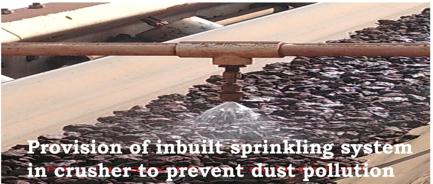
**Provision of inbuilt sprinkling system in crusher to prevent dust pollution**
