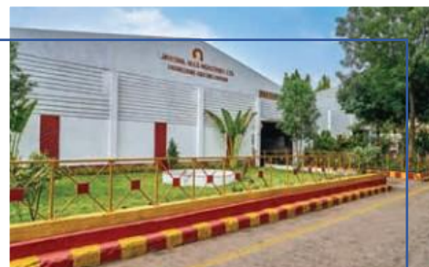
Engineering Castings Division, Nagpur
