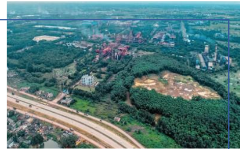
Integrated Steel Plant, Raipur
