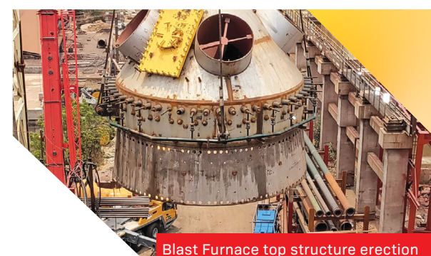
Blast Furnace top structure erection
