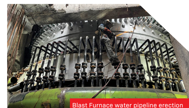
Blast Furnace water pipeline erection
